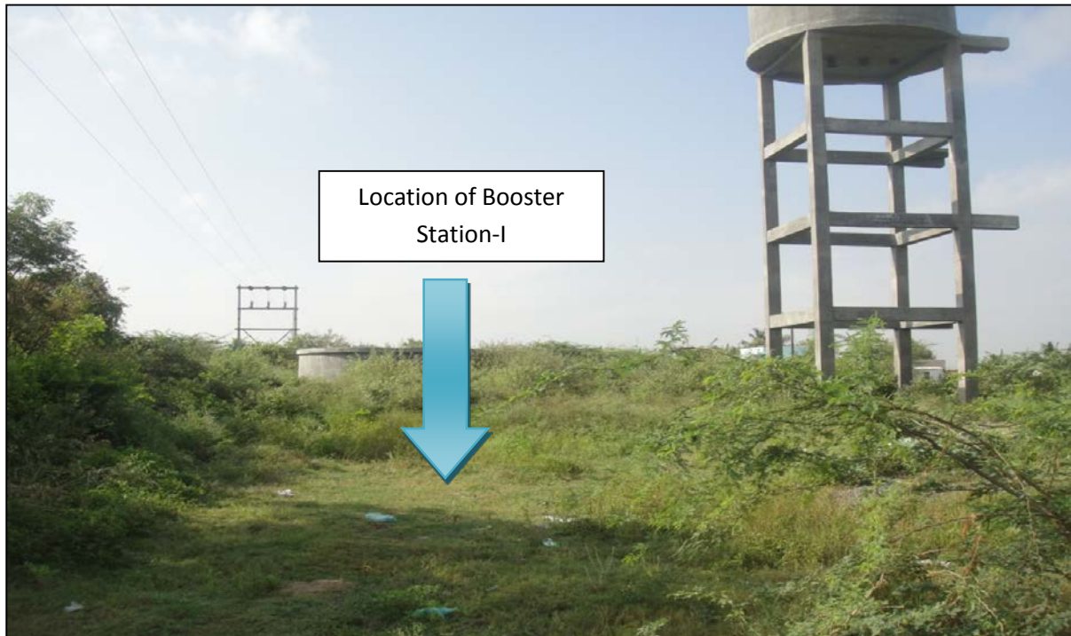
Figure 2. 4-Location of Booster Station - I at Manur
