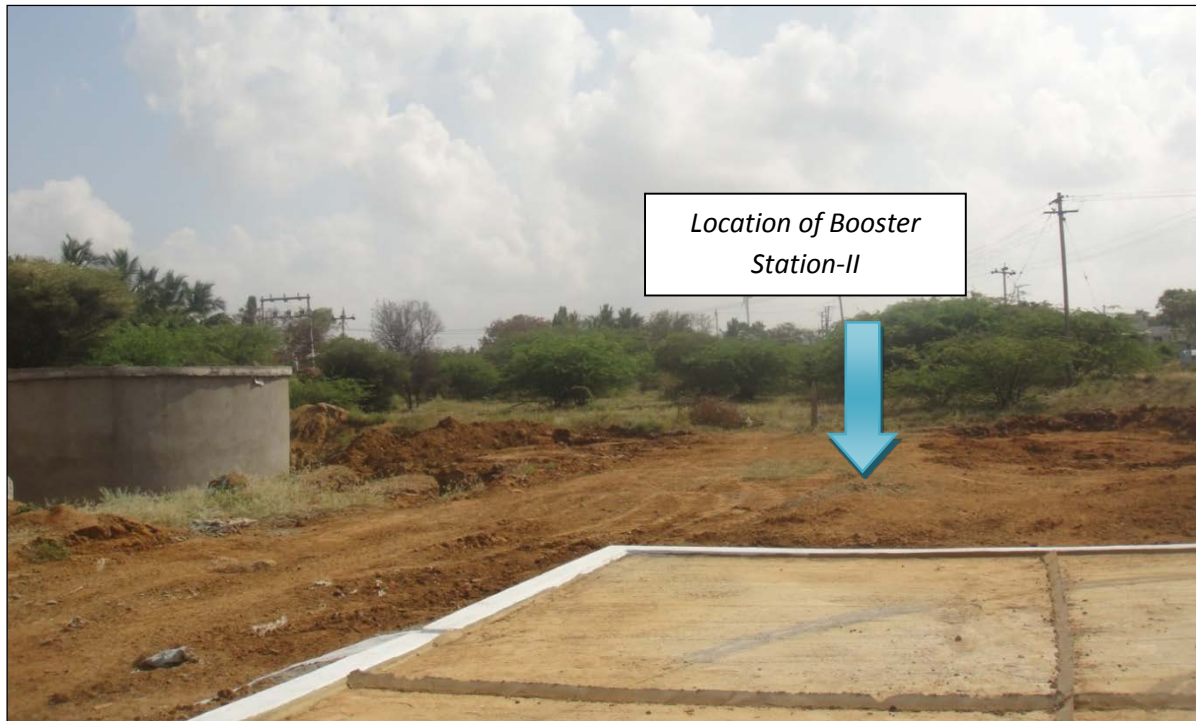
Figure 2. 5-Location of Booster Station - II at Panavadalichatram
